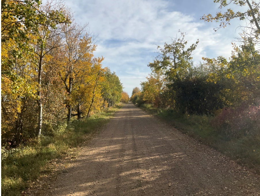
Appendix Photo D-3. View south within the Bypass footprint along Range Road 223, September 27, 2023.
