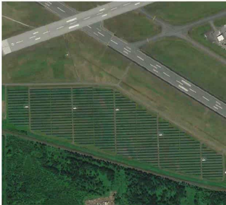
Thunder Bay Airport 8.5 MW Ground Mount Solar Completed 2011
