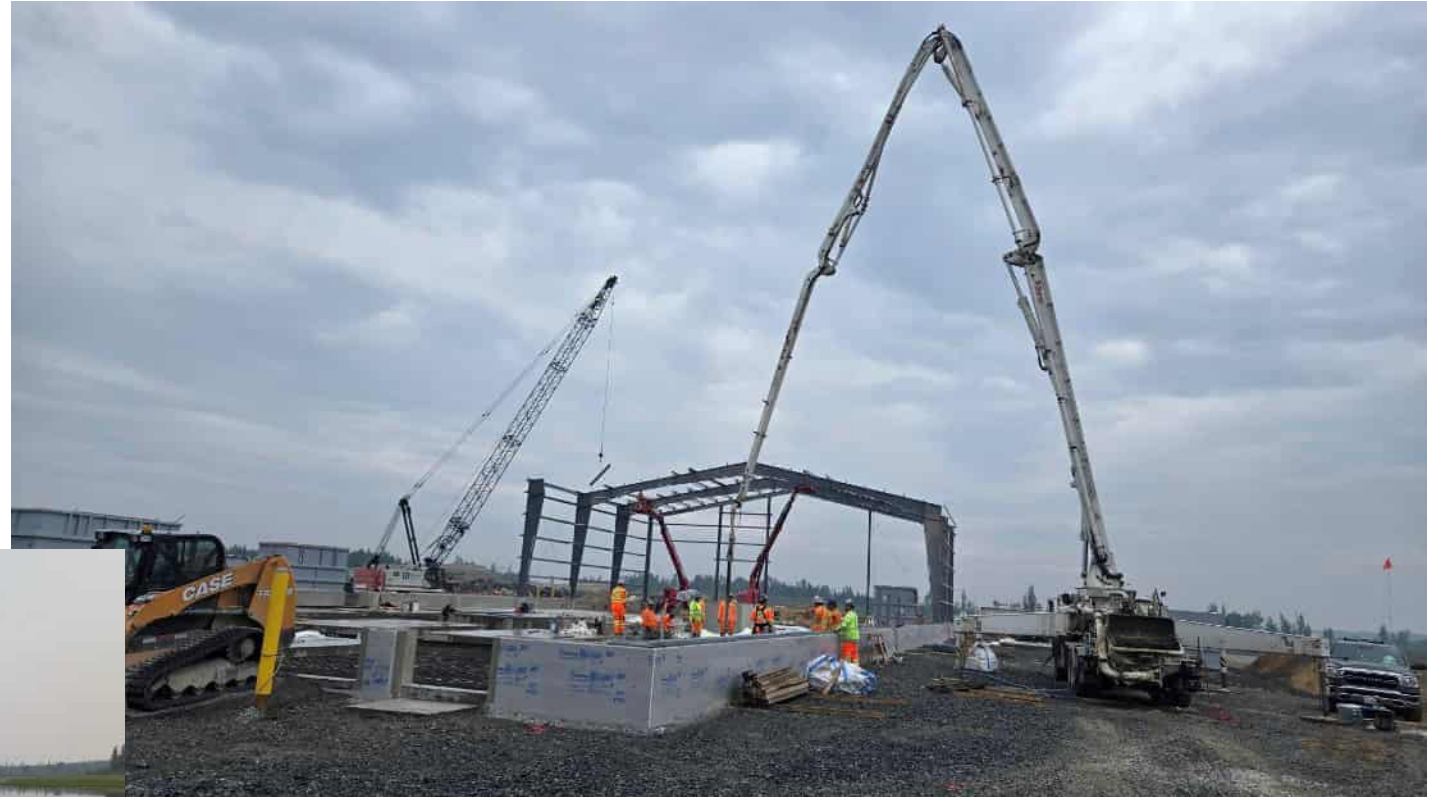
ETP Building Concrete and Steel Erection
