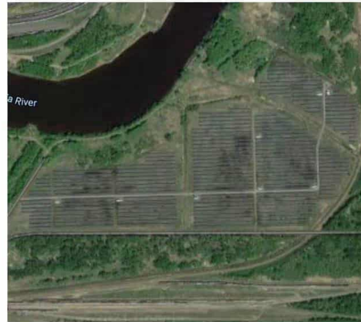
Fort William First Nations 10 MW Ground Mount Solar Completed 2011
