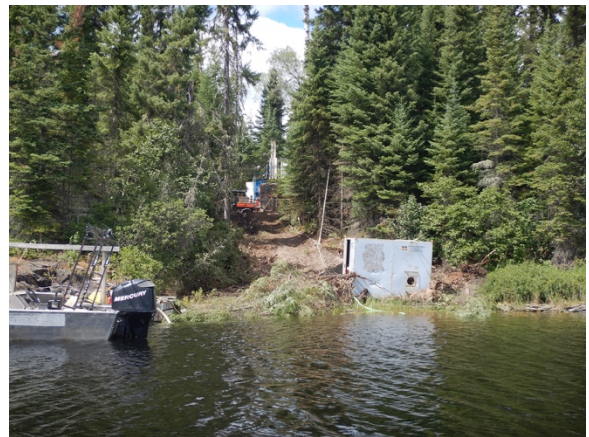
Figure 43: Disturbance, typical geotechnical drill site.
